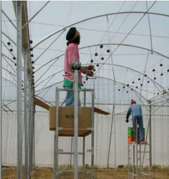
Trellising system assembly
